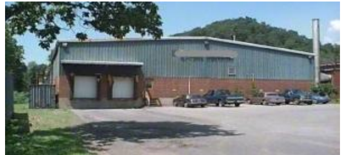
Figure 6 Warehouse Used for Prefabrication in Williamsport, PA
